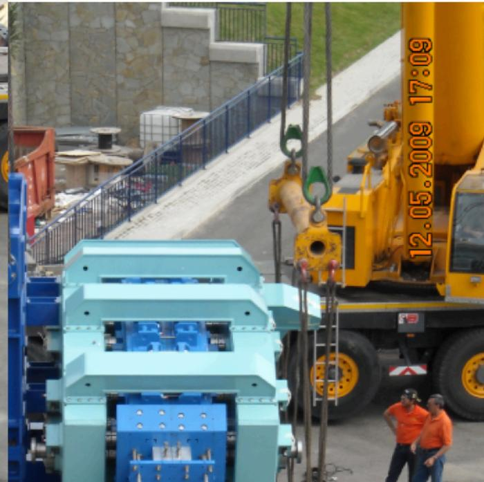
The CNAO 90° magnet during installation in the vertical line. The size is the same as for a gantry final magnet.
